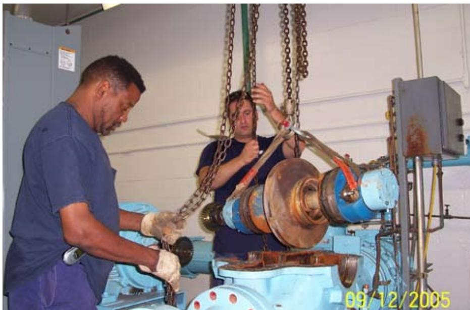
**Figure 1. Denise No. 2 horizontal split-case pump being taken out of service for repair and coating.**
